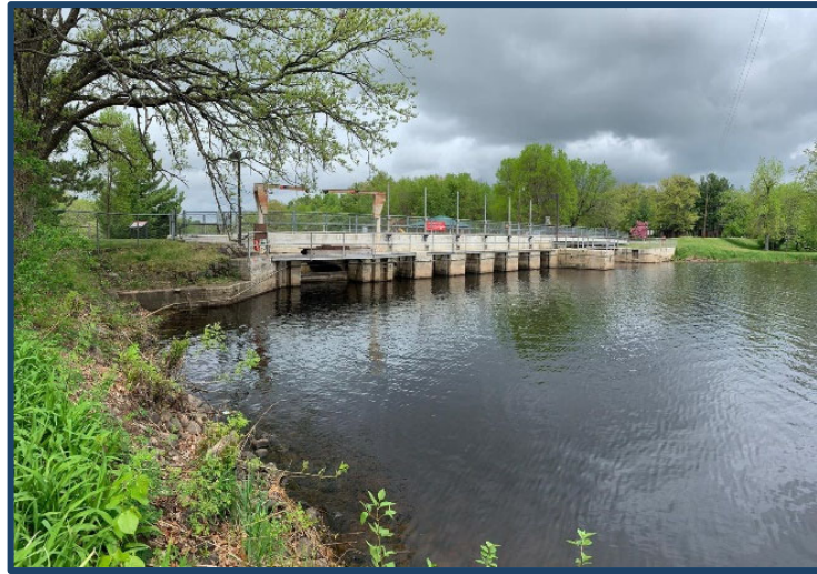
Figure 3.8 Sandy Lake Reservoir Lock and Dam.
